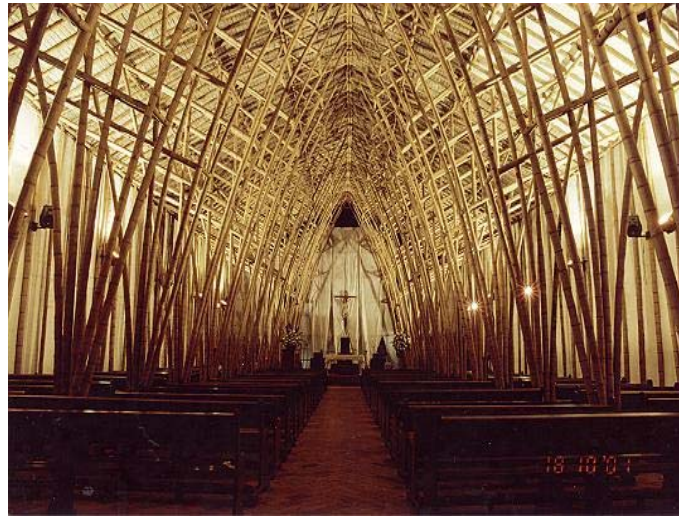
Church in Columbia by Simon Velez demonstrates the strength and versatility of bamboo – all well explained in Darrel's manual on Bamboo Building and Culture .
