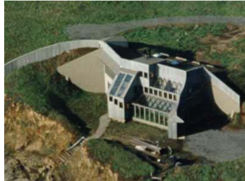
Heckerth residence in Mendocino, California, is all solar, requires no added heat, and its solar collectors also power the family's electric cars.
