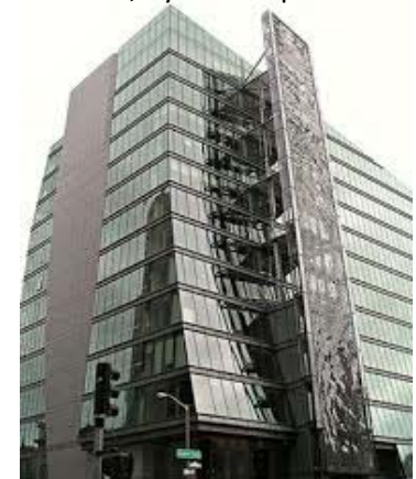
Wind power system for S.F. Public Utilities Commission building, by Reinhold Ziegler.
