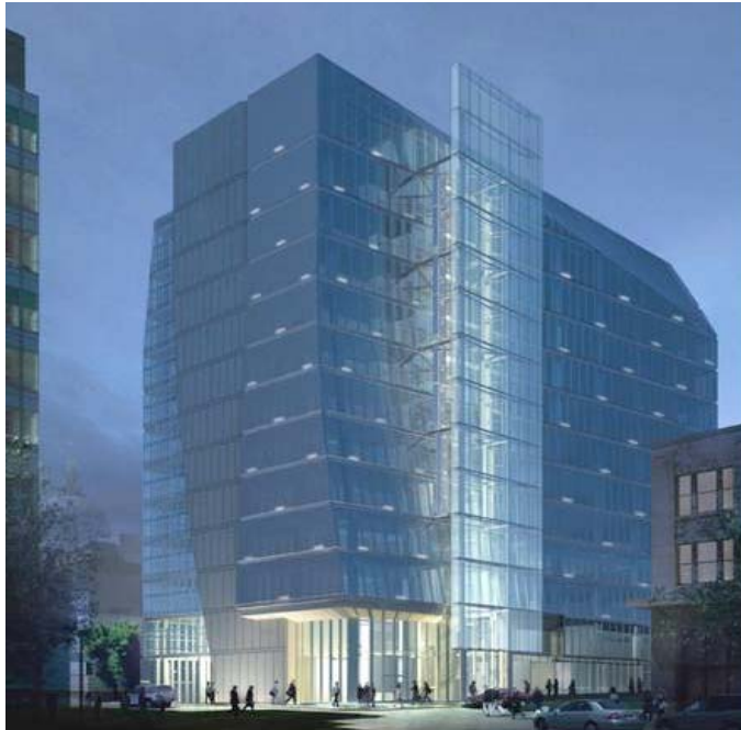
Wind energy system for San Francisco Public Utilities Commission building.
